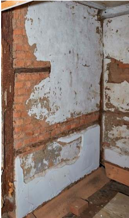
Figure 76. Detail of brick nog construction in Bedroom 4, ground floor. Source: Ross Thornton, 2019.
