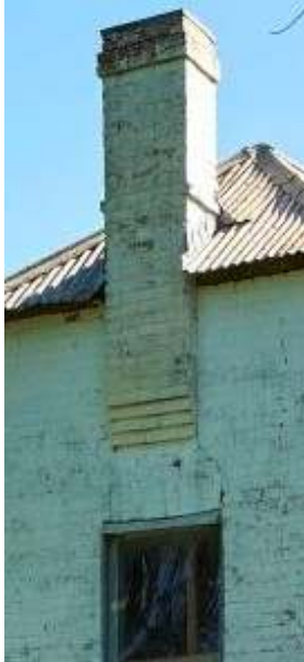
Figure 78. False chimney on south facade. Source: Ross Thornton, 2019.
