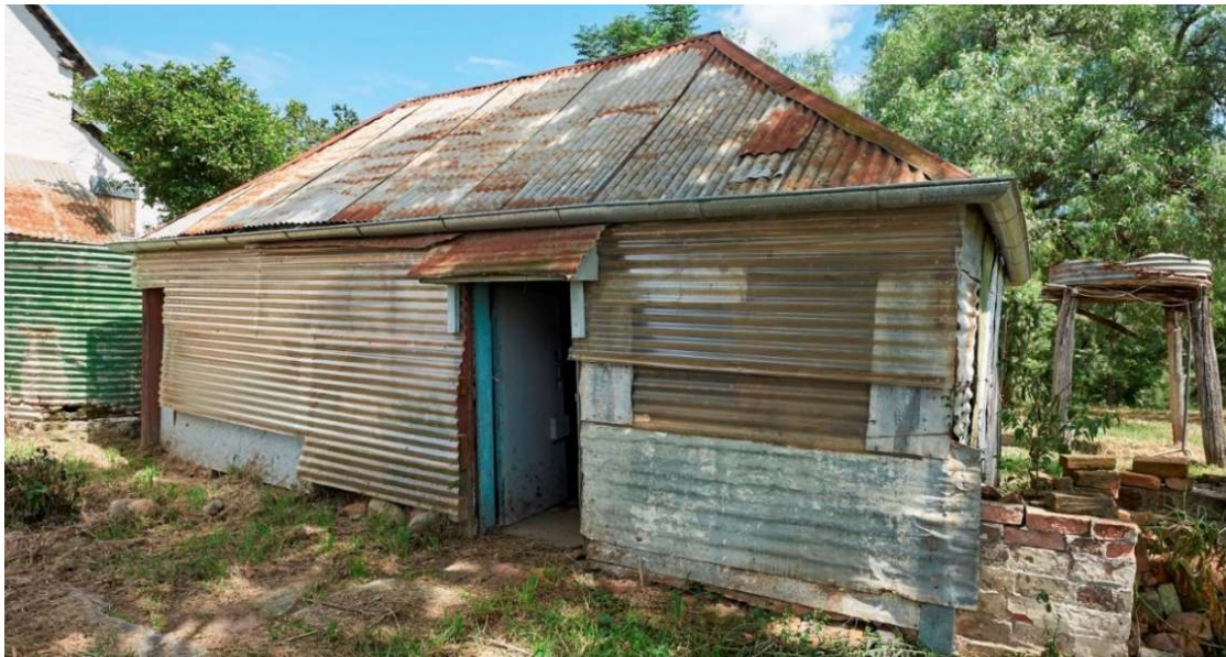
Figure 41. East elevation of the weatherboard cottage. Note the remains of the brick hearth and chimney at the right. Source: Ross Thornton, 2019.
