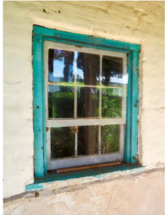
Figure 77. Unequal sashed window on ground floor. Source: Ross Thornton, 2019.
