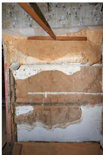
Figure 35. Wall in Bedroom 1 demonstrating brick nog construction. Source: Ross Thornton, 2019.
